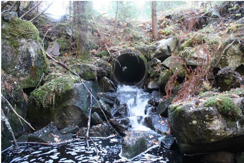
*Figure 8: Tributary B, Storrsjøbekken runs through a small pipe under a road. During normal water flow the pipe is possibly an obstacle for brown trout.*
